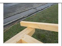
VISSAGE DES CHEVRONS (11) PAR VIS VBA 6 X 160 SUR SABLIERE POUR TERMINER
