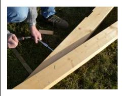
MISE EN PLACE DU TIREFOND POUR RENFORCER ASSEMBLAGE DE LA PIECE (10) AVEC PIECE (8) <u>Douille de</u> 17 mm
