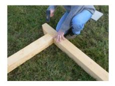
CHEVILLAGE DES ASSEMBLAGES NE PAS ENFONCER LA CHEVILLE COMPLETEMENT. ASSEMBLAGE POTEAU ET PANNE + VBA 6 X 200
